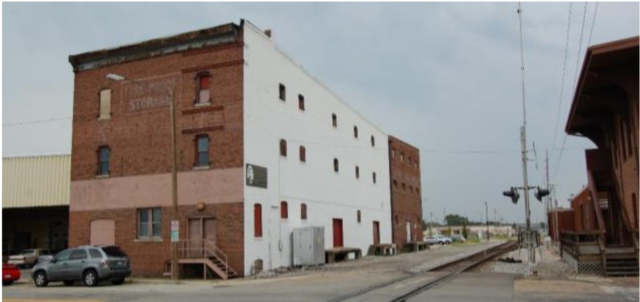
Former Fireproof Storage House No. 3 (No. 21) at left, 1000 E. Monroe Street
