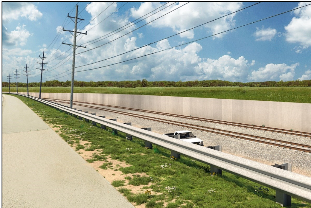
Exhibit D4-14. Rendering of Build Alternative 2A cut location with up to a 17-foot retaining wall west of UPRR (Station 2530+00)
